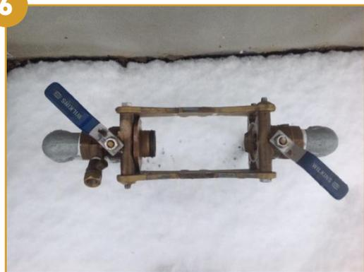
Re-open both ball valves 1/8 turn and leave them in a partially opened position to drain remaining water. Even a small amount of water left in the unit will freeze and could crack the housing.
