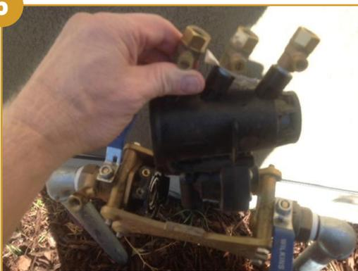
Remove the backflow body and store it in a warm place, but not in a garage.
