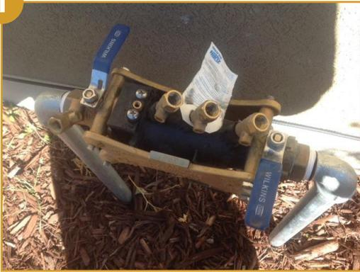
Turn off the main sprinkler supply. Then turn off the ball valves at both ends of the unit.
