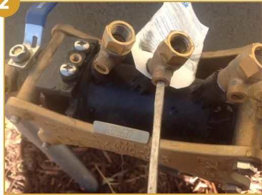
Twist the screw 1/4 turn on all three relief valves to bleed the pressure.
