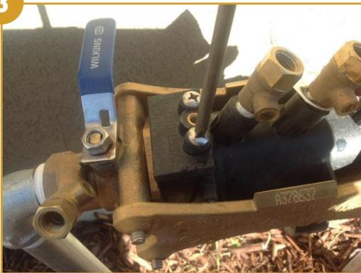
Remove the two screws on the top of the wedge piece.
